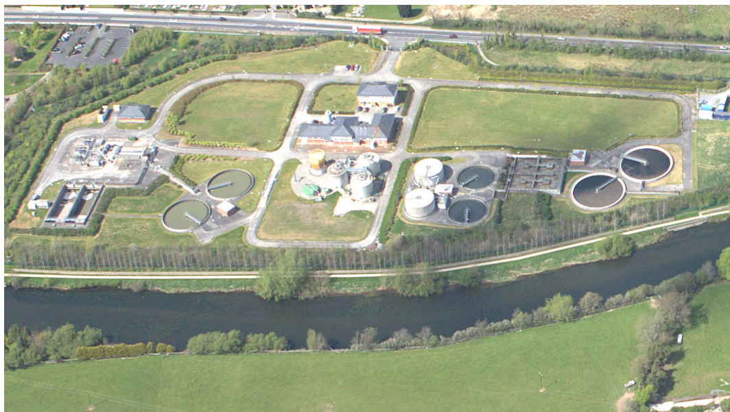
Clonmel Wastewater Treatment Works
