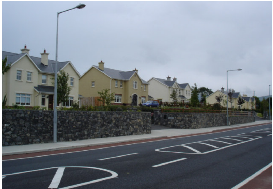
New cycleways on the Fethard Road
